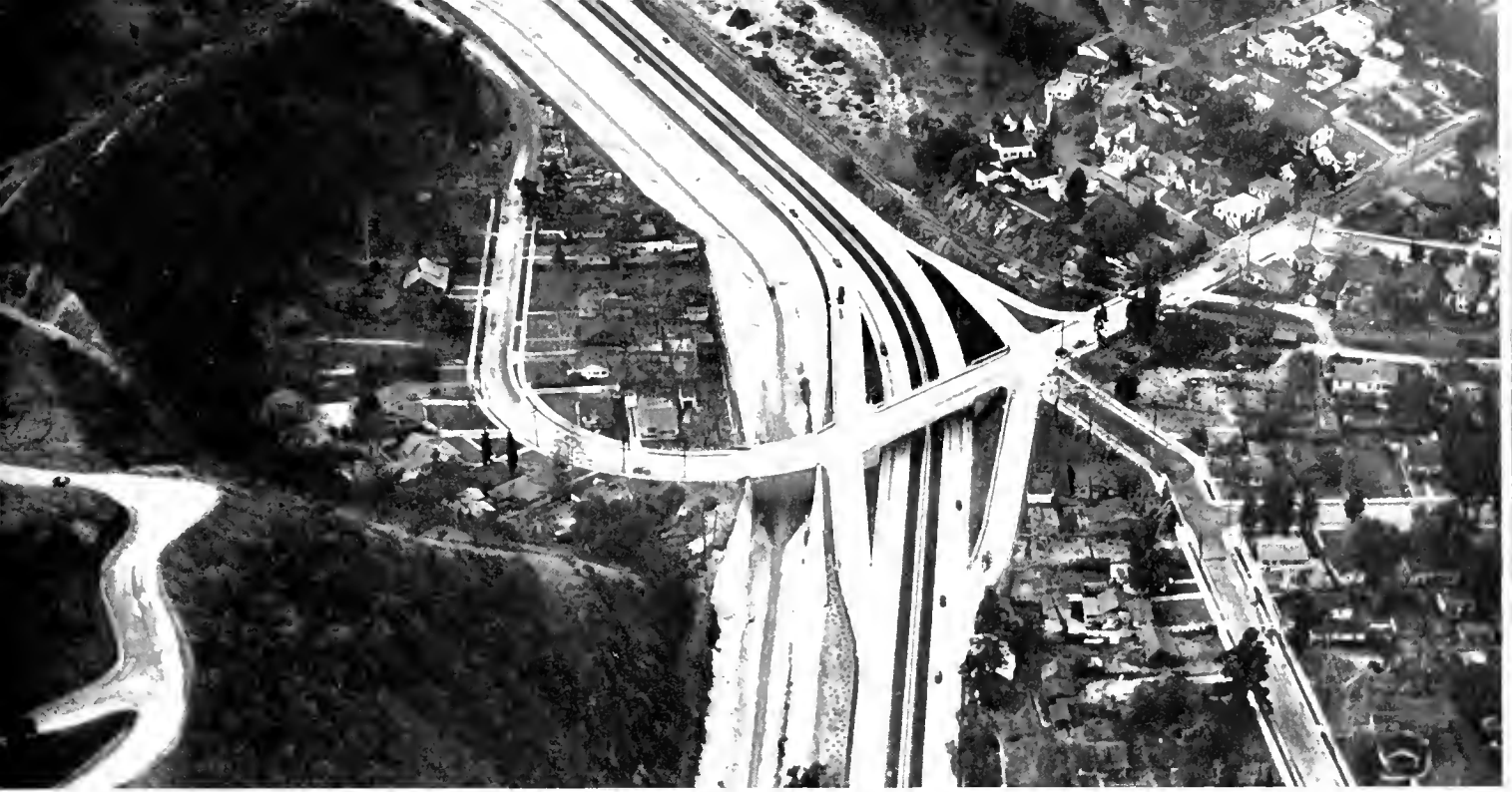
A multi-purpose structure involving problems of horizontal and vertical clearance, super elevation and intricate construction
